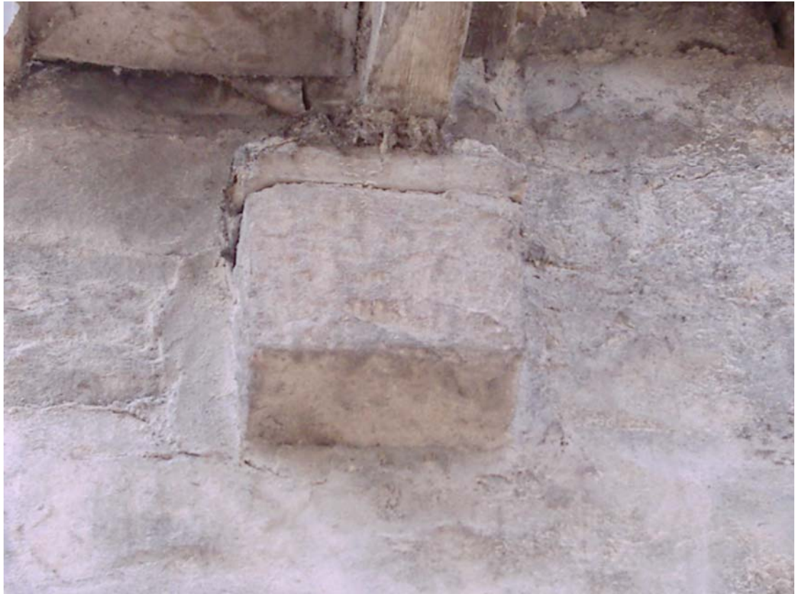
Plate 5: Stone corbel supporting the roof of the outshut
