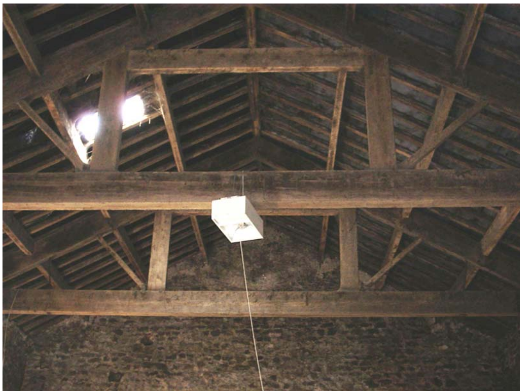
Plate 8: Detail of the queen-post and collar trusses
