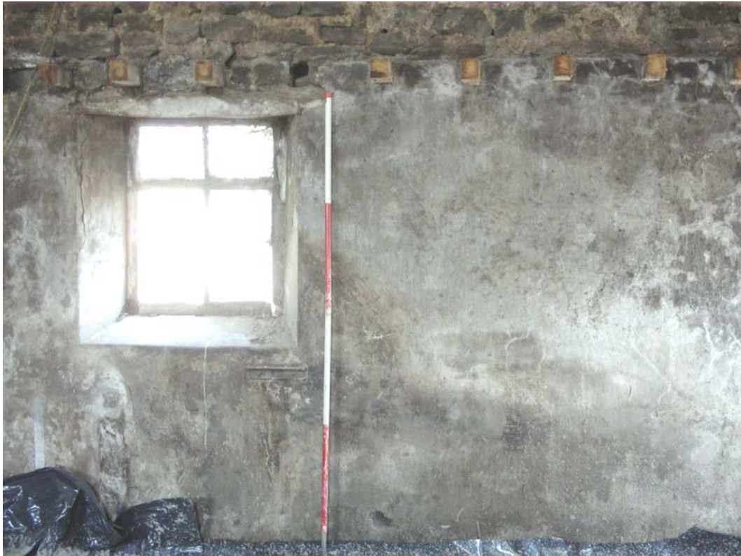
Plate 7: Detail of the interior of the windows and the remains of the hayloft at the east end of the barn.
