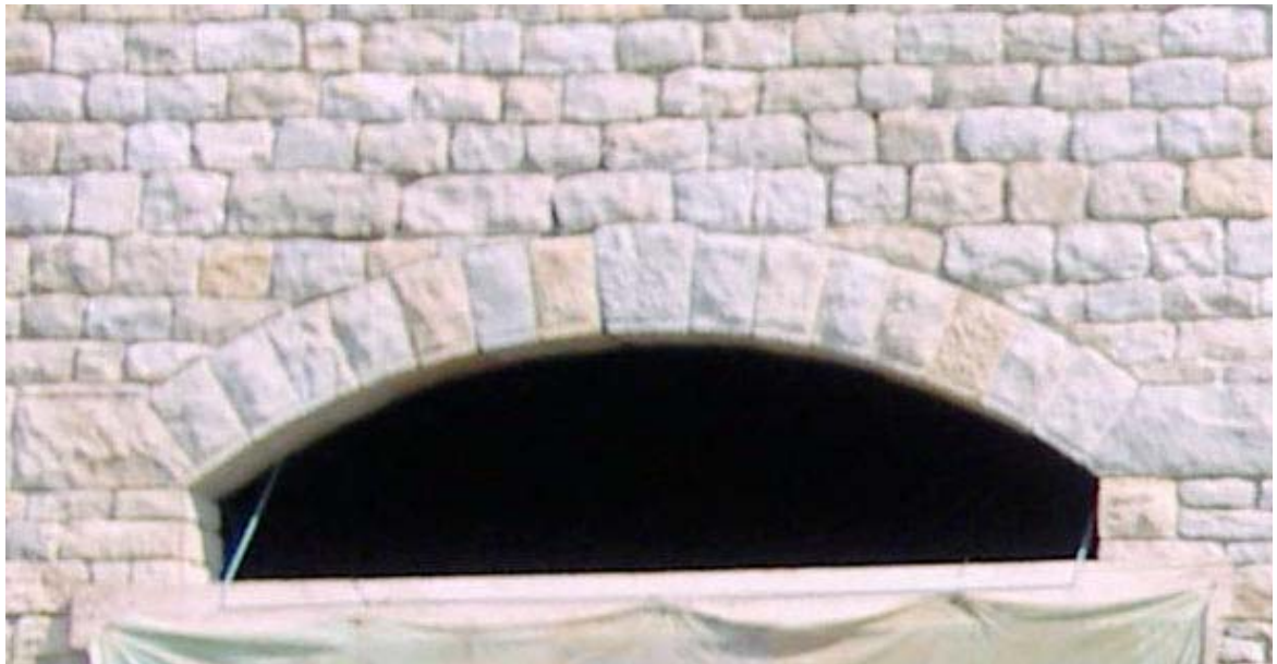
Plate 10: Detail of the well-fashioned voussoir around arch over the wagon doors
